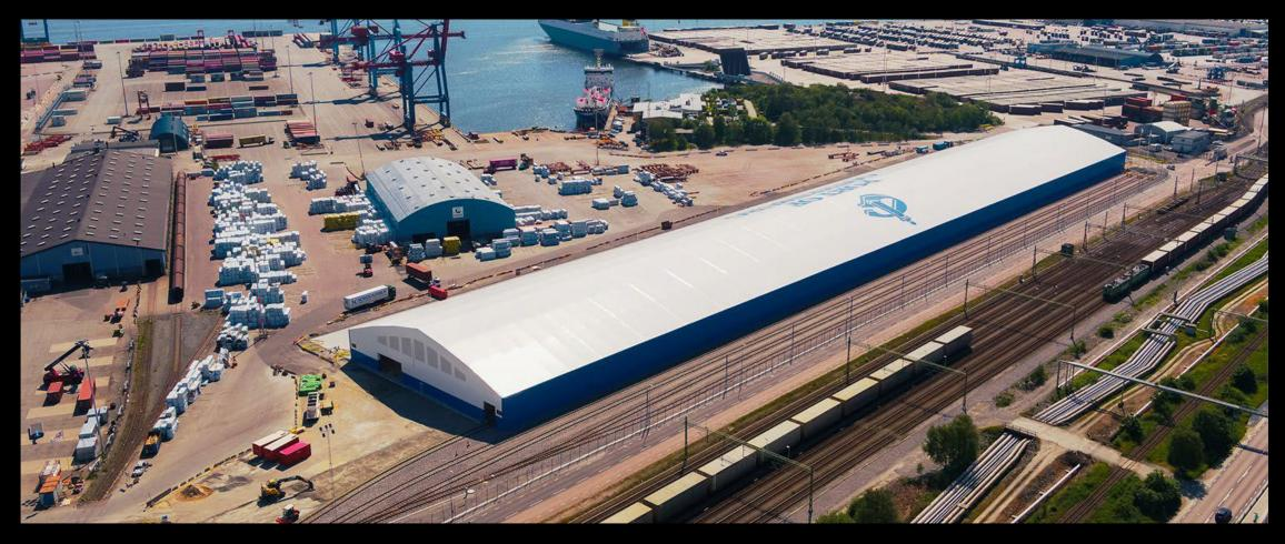
60 x 360 x 11m Clearspan structure 21.600 m2,
