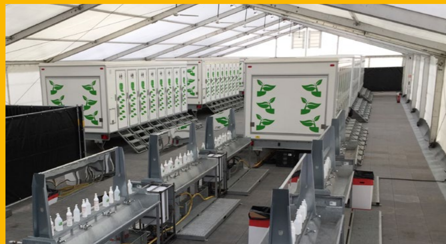
Toilets, showers, and hand washers
