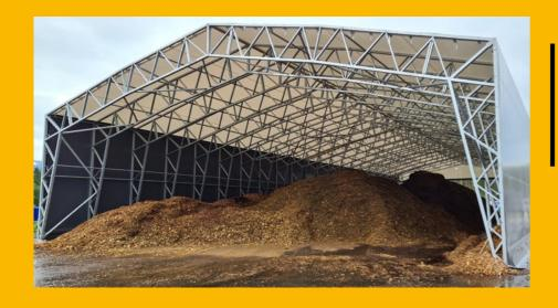
In most cases, these structures do not require extensive foundation and can be anchored directly to the ground.
