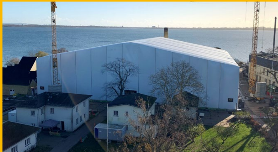
Giant Weather Shelter On rails 65x50m, 13m height
